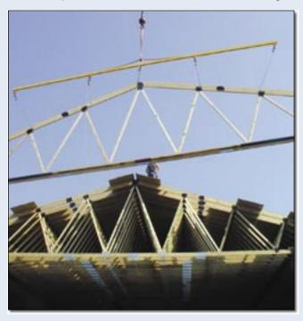
STEP 8: Repeat steps 6 and 7 with the remaining trusses using the sheathing each time as both the temporary and permanent bracing. This approach can result in a fully sheathed and permanently braced roof system in the same time it takes to install the trusses with only temporary bracing.
