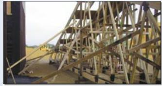
STEP 3: Brace webs laterally and diagonally where required by the Truss Design Drawing. Install bottom chord permanent lateral bracing every ten feet, and
