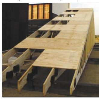
**STEP 4:** The first set of five trusses is the "superstructure" which provides a solid foundation to laterally support additional trusses.
