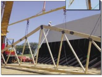
**STEP 6:** Install 4x8 sheathing in the alternating gaps so that two feet extends past the sixth truss. Fasten the sheathing to trusses per construction documents.
