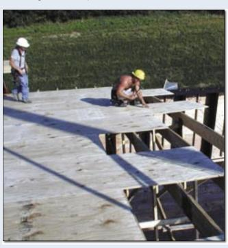
**STEP 7:** Hoist the seventh truss into place and attach the sheathing to the top chord. At the same time, the crew can install the permanent web and bottom chord bracing.
