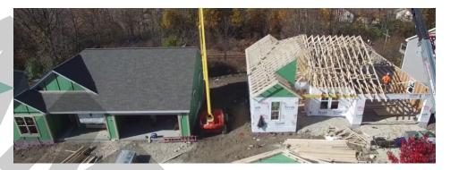
The only difference between the two homes was one house was entirely stick-framed, while the other home was framed using structural components, including roof trusses, wall panels and floor trusses.
