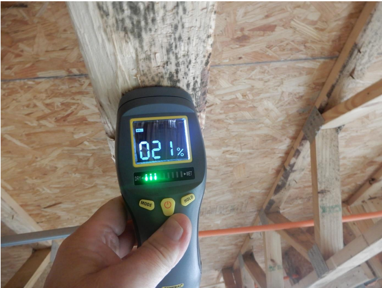
Photo 3: Wood Tested with Moisture Meter
