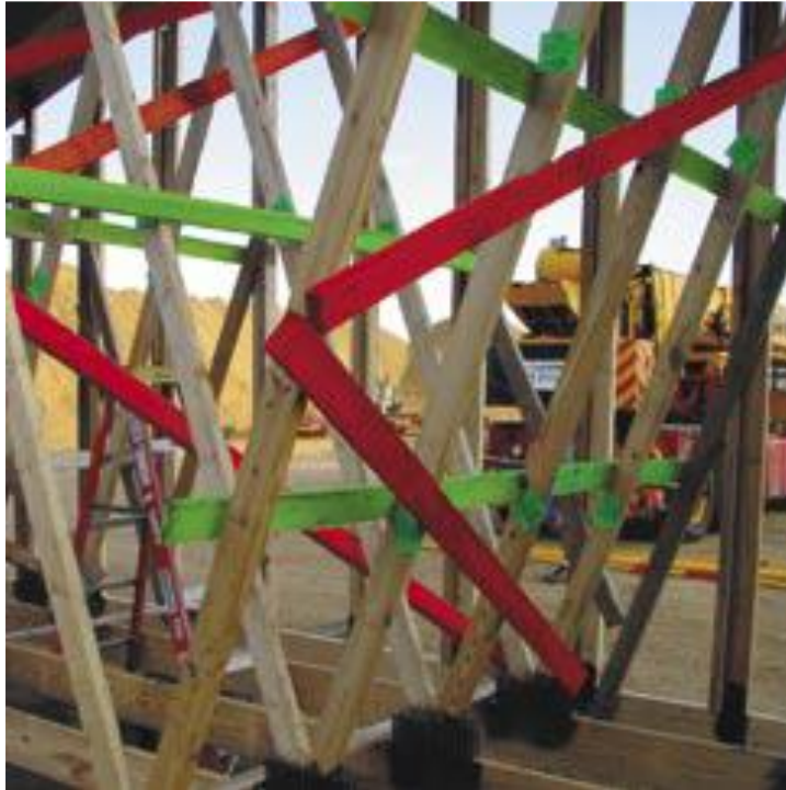
Photo 3: Diagonal/Lateral Web Bracing on First Five Trusses as Specified
