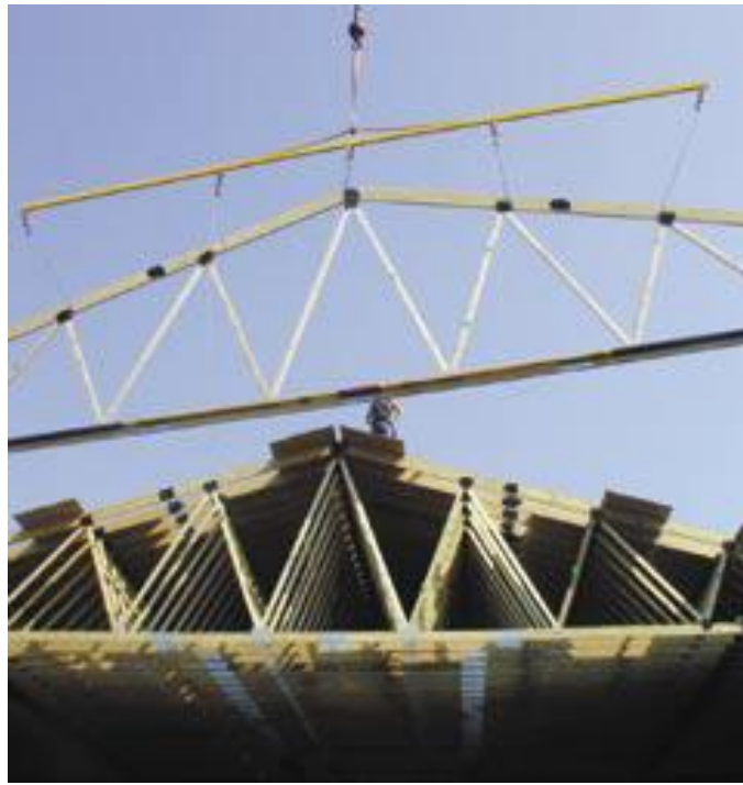
Photo 7: Hoisting the 7 th Truss
