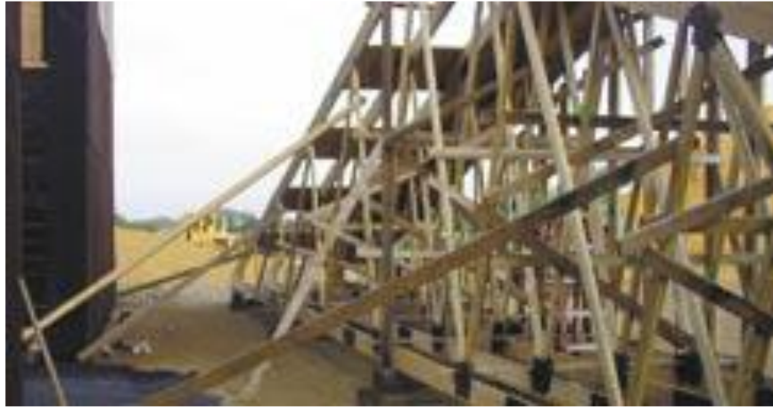
Photo 1: Ground Bracing on First Five after Bearing Timbers are Levelled
