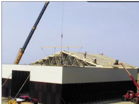
Photo 8: Installing and Bracing Each Truss
