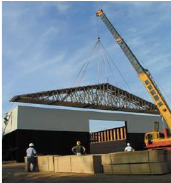
Photo 4: Raising of “Superstructure” Set of Trusses off Ground
