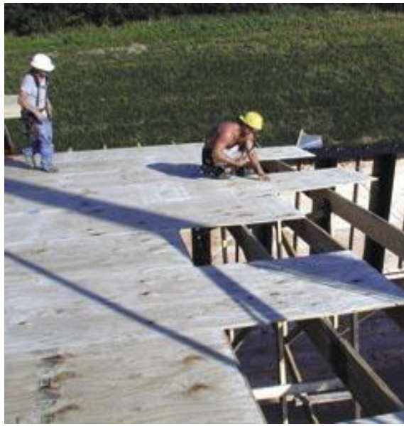
Photo 6: Installation of Top Chord Sheathing as Trusses are Installed
