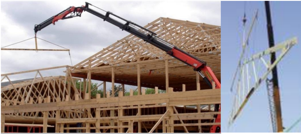
Photo 5: Spreader Bar Attached to End of Crane for More Rigid Hoisting
