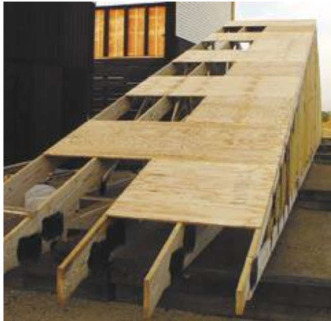
Photo 2: Sheathing on First Five with Alternating 4x4 and 4x8 Sheets
